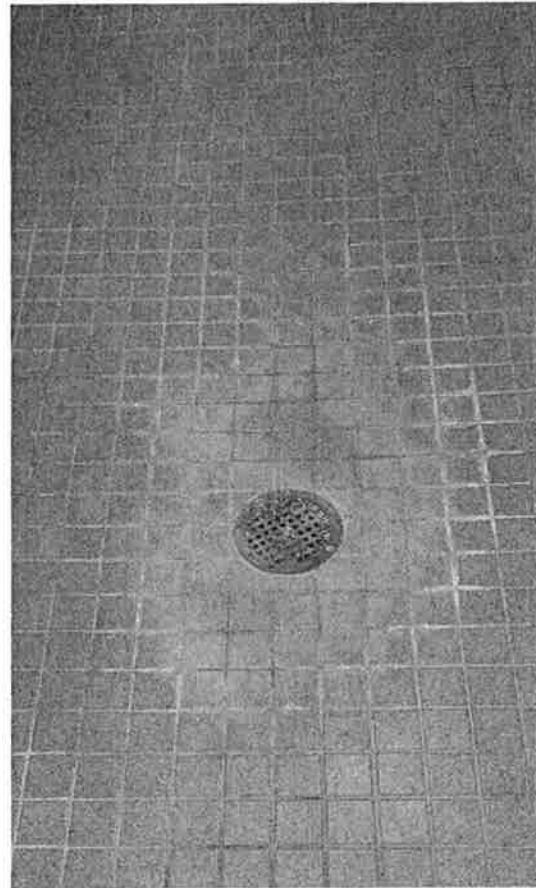
Shower drain repair caused by destabilization of slab
