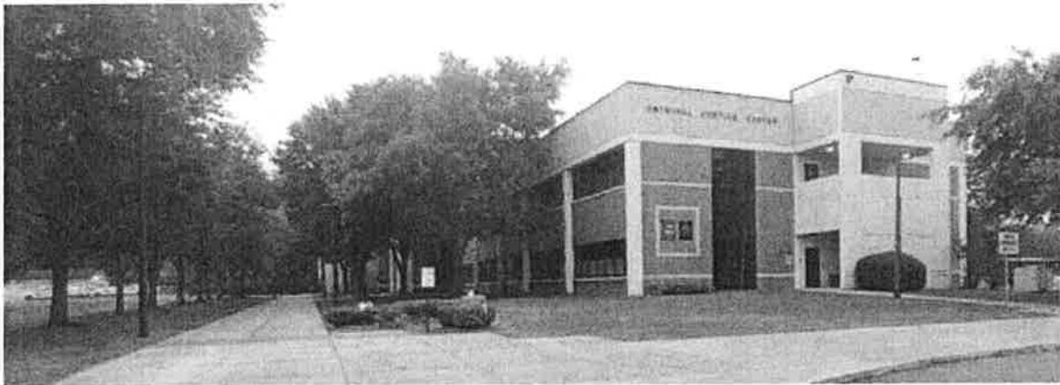
Criminal Justice Center, Building P, North Campus
